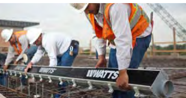
Water Re-use & Drains
