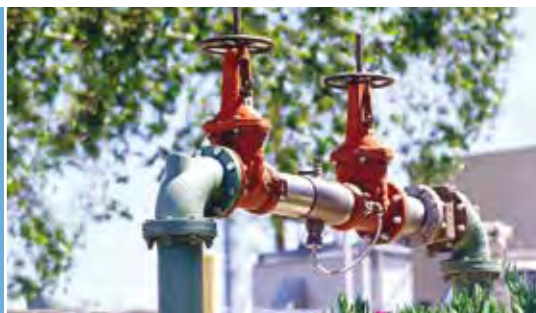
Plumbing & Flow Control
