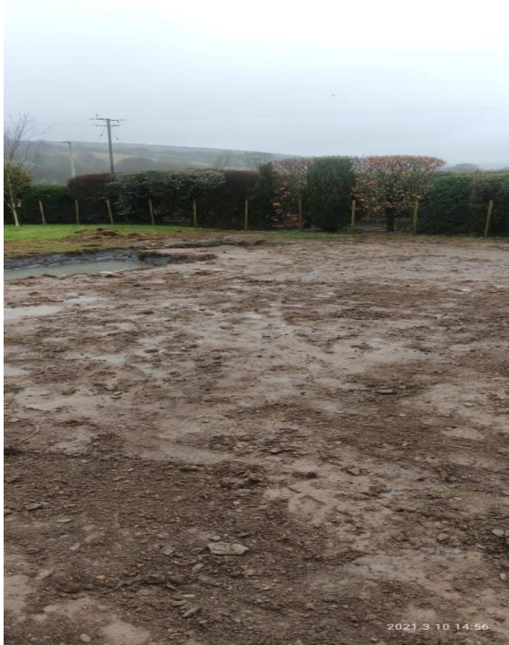
Area after re-instatement by the ground work contractor for a large 5 borehole system.
