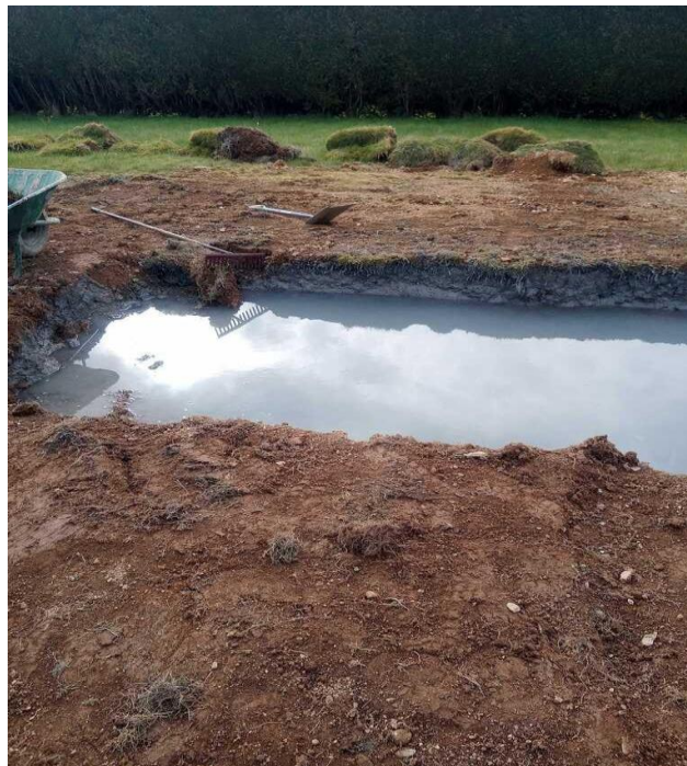
Customer prepared a sump to take water from the boreholes preventing running into adjoining property, this will gradually empty.
